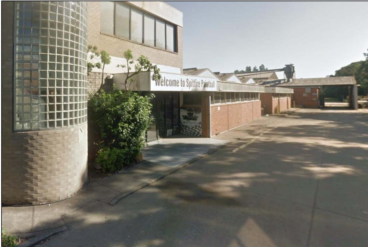
Plate 1 Existing warehouse located on-site (brick construction so would afford a significant impediment to flow) (Google, 2018)
