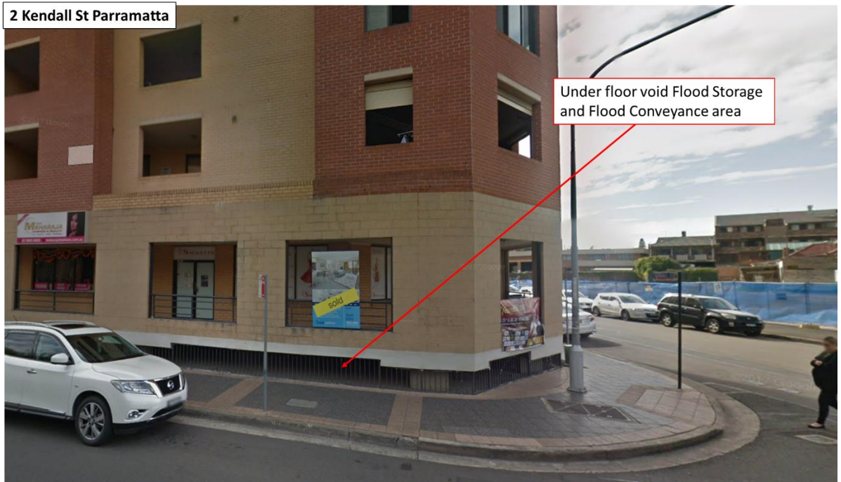
Plate 9 Example of under floor void flood storage and conveyance (2 Kendall St Parramatta)
