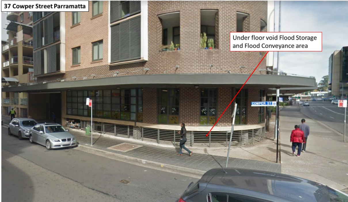
Plate 6 Example of under floor void flood storage and conveyance (37 Cowper St Parramatta)
